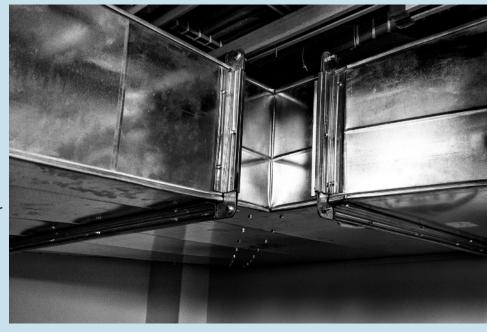
look at it, your system is not functioning as it should and you're losing comfort and money. The purpose of an HVAC system is to move heat, not waste it. If sealing duct leaks and other repairs (crushed or open ductwork, closed or broken dampers, undersized returns, etc.) cause an increase in static pressure, affecting overall CFM, other measures should be taken to correct the static pressure problem. This is what separates good contractors from all the others.
